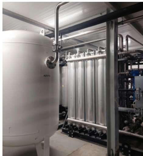
Amkor Portugal installed heat recovery and nitrogen production systems.
