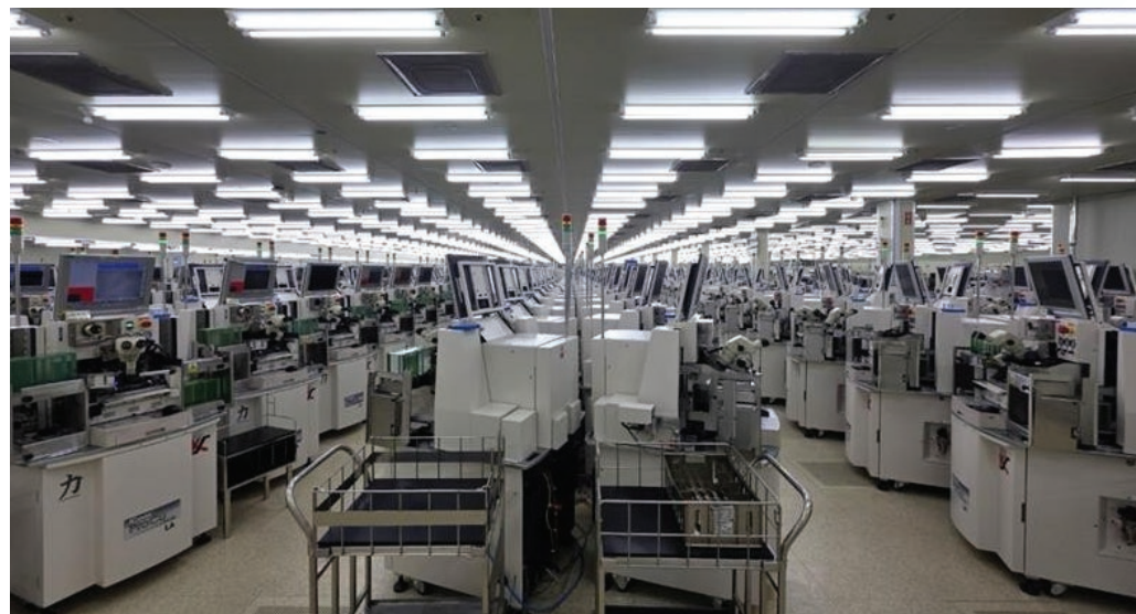
Energy efficient equipment and LED upgrades implemented at our South Korea site.
